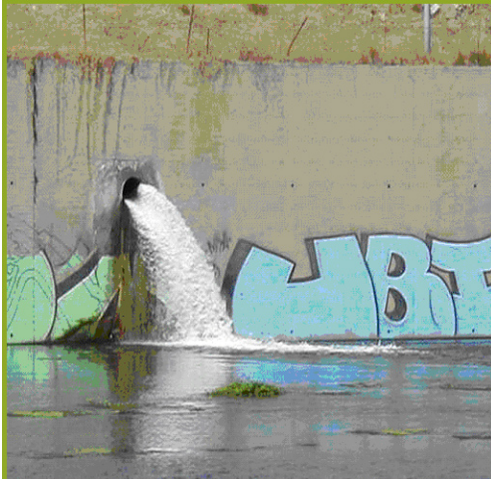
Photo 1 Glendale Los Angeles River Water Reclamation Plant Effluent Outfall (CRWQCB- LAR 2007a)
